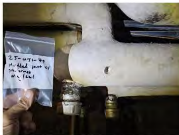
Photo #8 Photo of asbestos containing TSI mudded fitting with Mag/Cal pipe insulation, HA 25.
