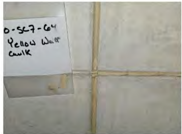
Photo #6 Photo of asbestos containing yellow wall caulk, HA 20.
