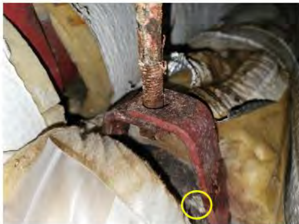
Photo #3 Yellow circle indicating asbestos-containing residual white thermal system insulation (TSI) mudded fitting on fiberglass pipe, HA 17.
