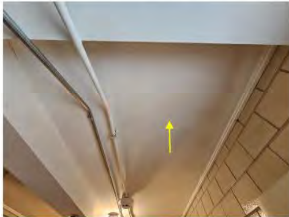
Photo #1 Photo of asbestos containing material (ACM), white plaster, homogenous area (HA) 01.
