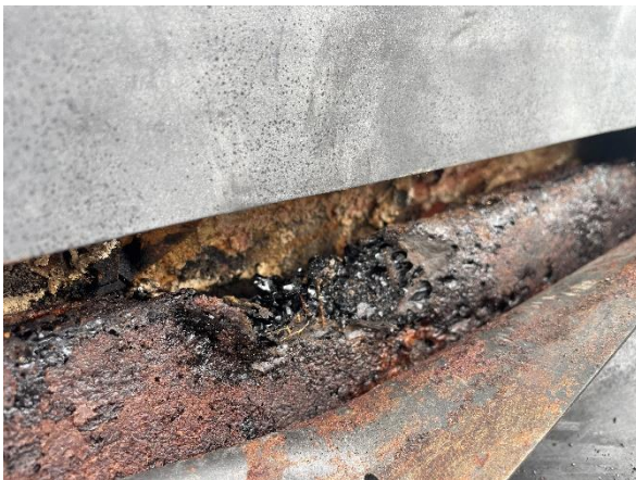
Photo #3 ACM Sample #6 Parapet Wall, base material (black) – 15% Chrysotile
