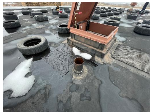
Photo #5 Small Roof Vent Penetrations and Hatch
