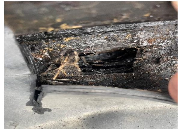
Photo #6 ACM Sample #7 Roof Penetration, base material (black) – 15% Chrysotile
