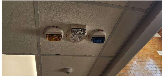
New notification devices at recent renovation for hearing impaired students
