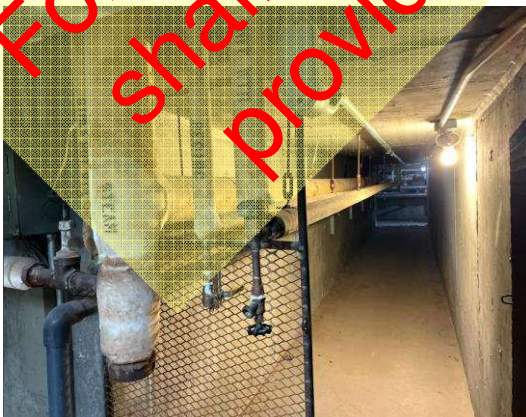
Domestic heating water and steam piping from utility tunnel
