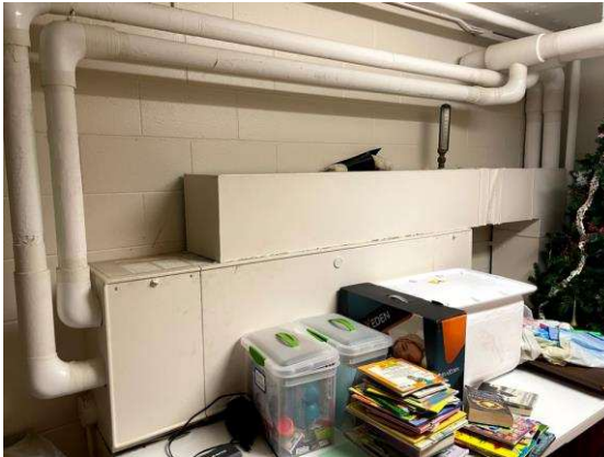
Fan coil serving basement lobby C110
