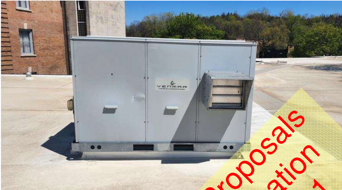
ERV on roof of new wing
