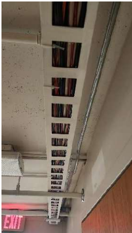
Cable Tray with numerous cable types bundled together
