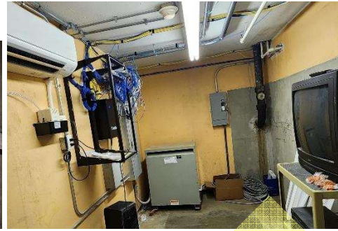
Existing IDF with Newer cabling
