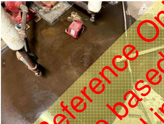
Clogged floor drain in mechanical room M103
