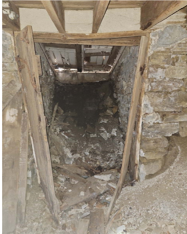
BASEMENT CELLARWAY - EXTERIOR STAIRS & SAGGING SILL BEAM
