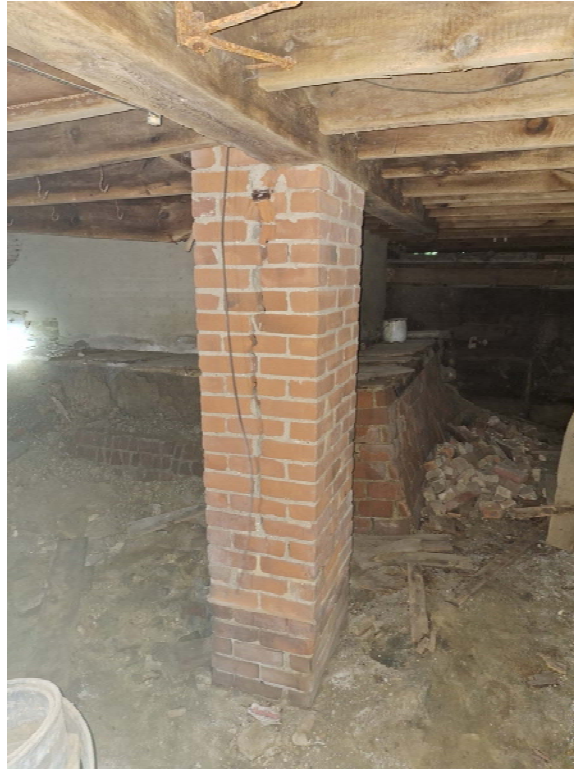
BASEMENT CHIMNEY - LOCATION OF BRICK CRACK REPAIR AND NEW SUPPORT POSTS
