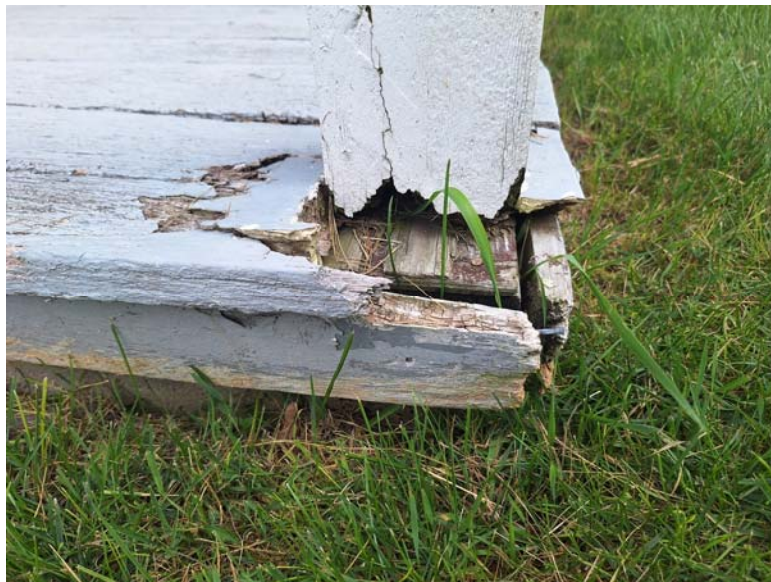
PORCH COLUMN AND FLOOR REPAIR
