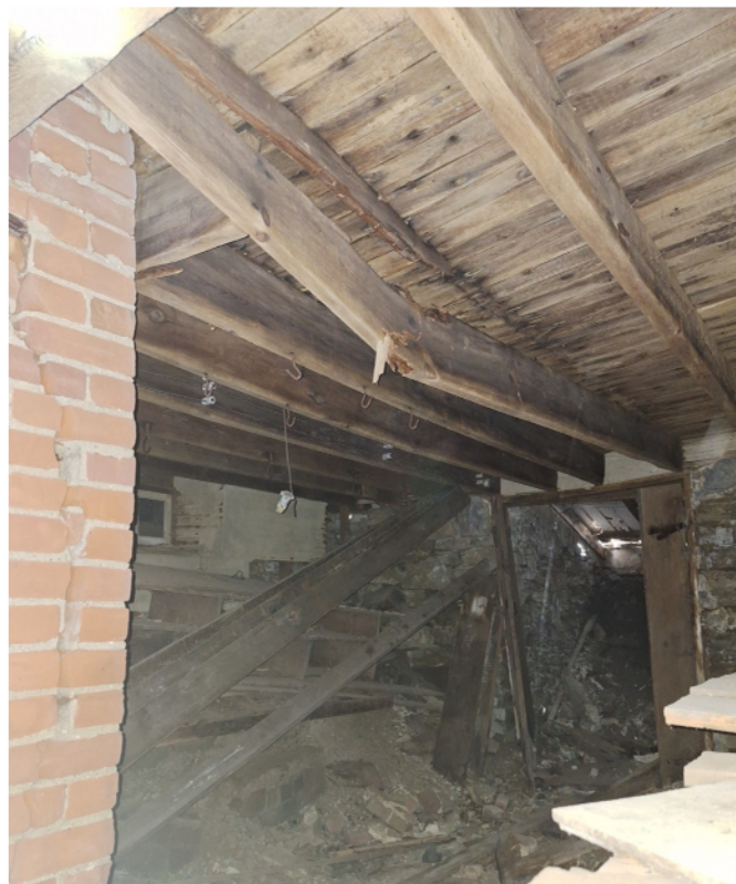
ROTTED FLOOR JOISTS AND FLOORING
