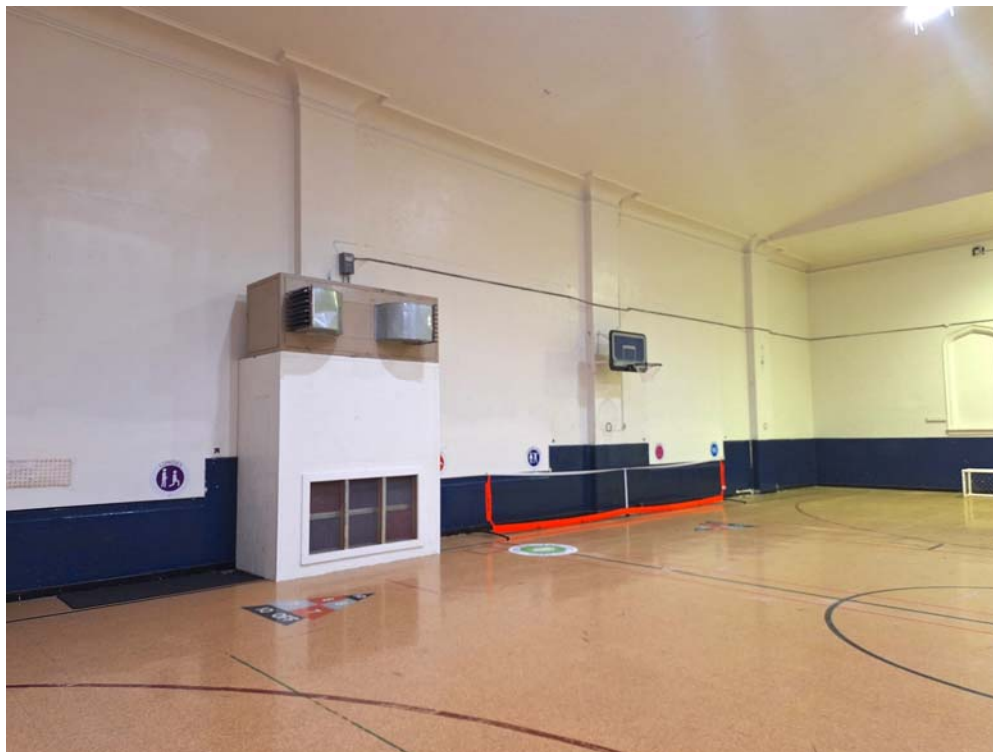
EAST WALL HEATING TO BE REMOVED
