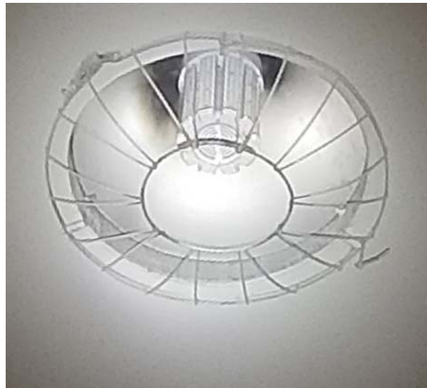
EXISTING GYM CEILING LIGHTS TO BE REPLACED
