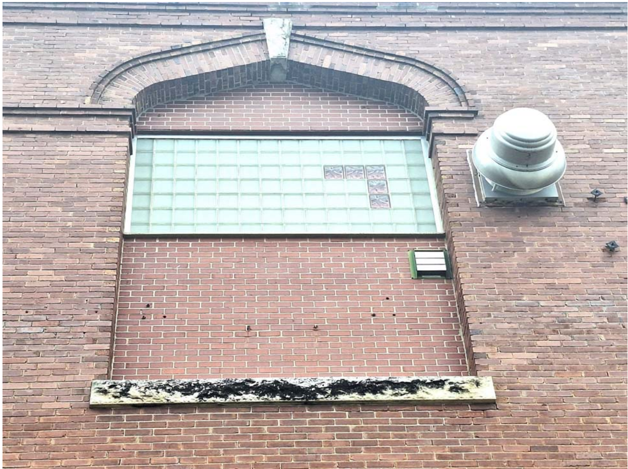
WEST EXTERIOR WINDOW INFILL TO RECEIVE HVAC LOUVERS AND LINTELS
