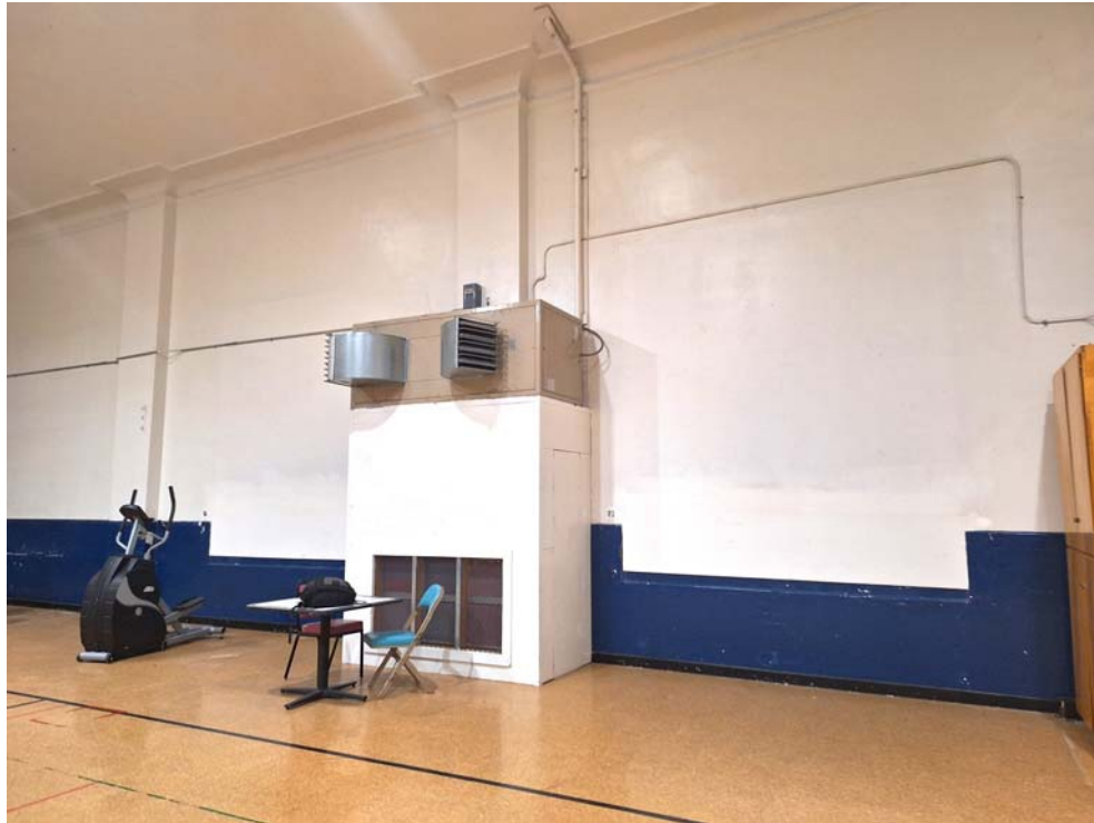
WEST WALL HEATING TO BE REMOVED
