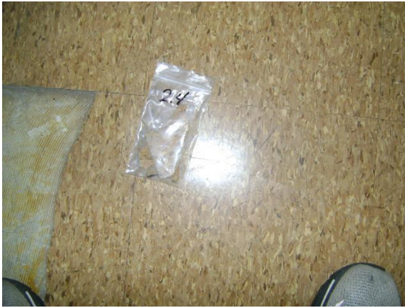
Photo #1 Asbestos containing floor tile (gold w/brown & white confetti) – CMHI Gym (2% Chrysotile)
