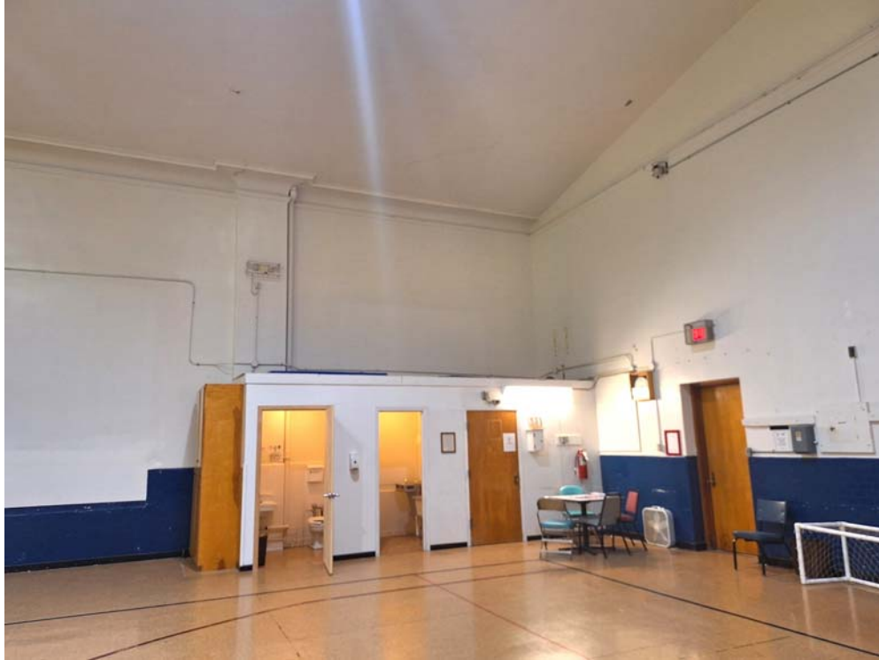
WEST WALL RESTROOM AND UTILITY ROOM
