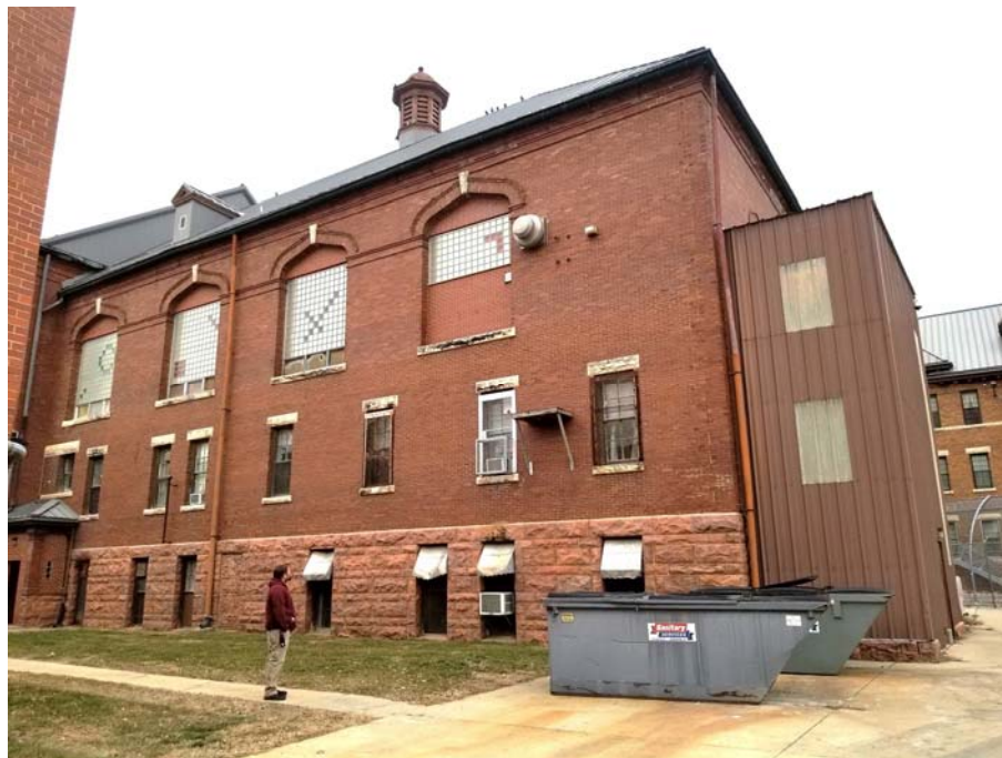
GYM EXTERIOR - VIEW OF WEST WALL
