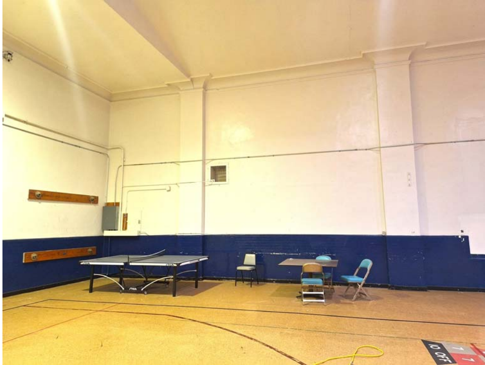
WEST WALL LOOKING AT AREA FOR NEW HVAC UNIT INSTALL
